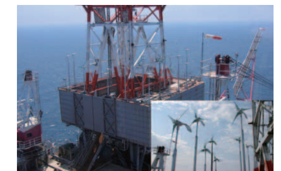
Twenty one Airdolphins form an AC power micro-grid on an unmanned offshore gas rig.
