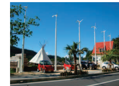
Electric Car Plug-in Charging System
